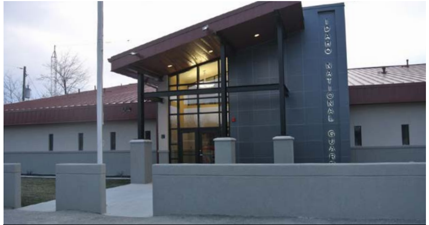
The Emmett Readiness Center was renovated in 2015.
