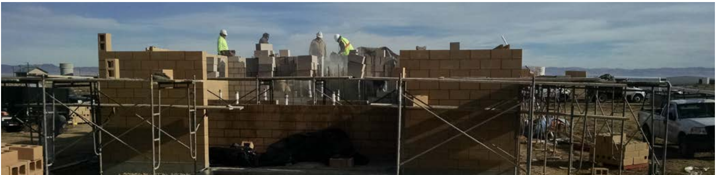
Construction in the cantonment area at the Orchard Combat Training Center is scheduled for completion in February of 2016.
